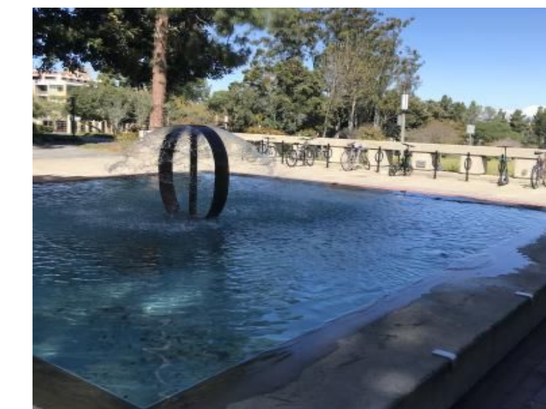
Figure 5: UCI's Infinity Fountain overflowing after rain
